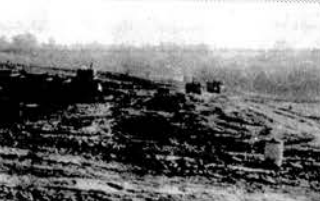
Loudon. Site preparation will take another month and will be followed by the construction of the large plant. When completed the facility will employ some 350 persons.
