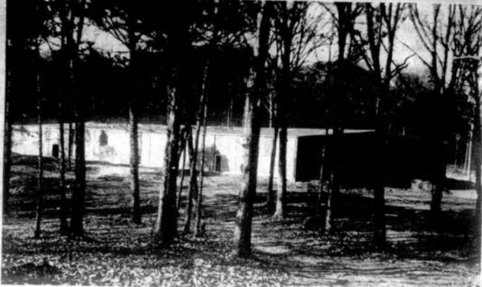
CONSTRUCTION CONTINUES on the new Loudon Sportswear plant on Carding Machine Road. The large steel and brick building is expected to be complete in the
