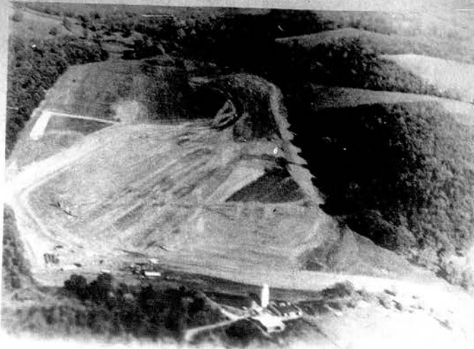
SITE PREPARATION CONTINUES at Loudon on the Ralston Purina Mushroom Farm site. Work on the plant itself is due to begin next month. The facility is being
