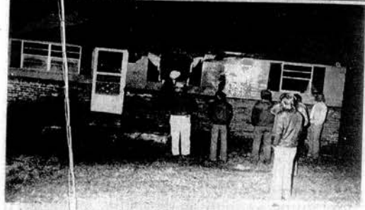
HOME DAMAGED —The home of Frank Coker, Jr., Grimes Road, Loudon, was heavily damaged by fire about 8 p.m. last Friday night. The Loudon County Rescue Squad extinguished the fire and saved the house from destruction.
