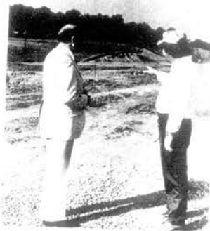
Stafford discusses construction on Highway 95 with Wayne Rollins Foreman for M. C. West Inc.
