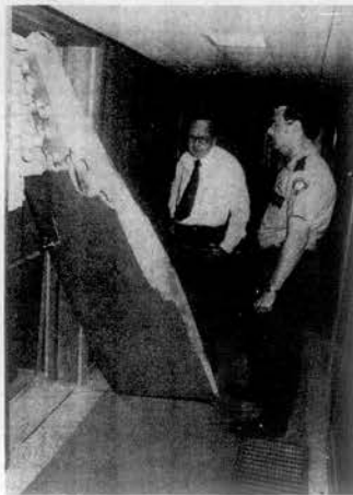
Deputy Allen Clemmer is shown in the church office looking at damage. Rev. Otis Campbell and Clemmer look at a door the thieves broke down to reach the main floor of the church. The thieves used candles for light while in the church.
