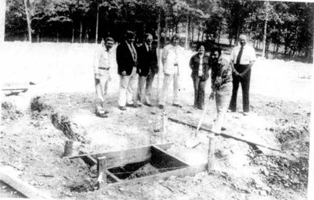
GROUND BROKEN FOR NEW PLANT—Tony LeSelva president of Loudon Sportswear, Inc., turns the symbolic first shovel of dirt at the official groundbreaking of the firm's new 20,000 square foot plant on Carding Machine Road in the Loudon Industrial Park. Pictured, left to right are: Bart Liddins, county industrial agent; County Judge
