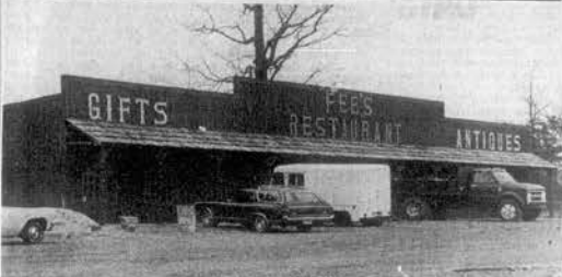
FIRST AT 72 AND 75 INTERCHANGE —A restaurant and gift shop known as Fees is under construction at the I-75 and State Route 72 interchange at Loudon. The owner, H. C. Fee, says the business, which will also sell gasoline will open probably in February. He stated the business will be keyed to local trade as well as tourists.
