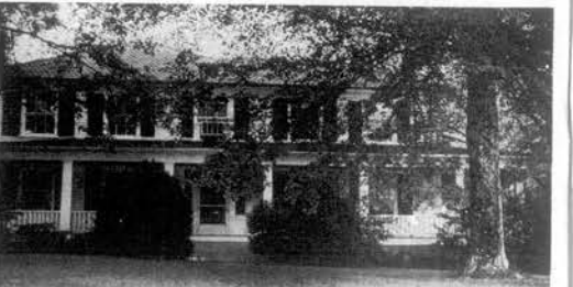
THE EUGENE ARMSTRONG, home on Martel Road, is believed to have been built by Reverend John Grant, a son-in-law of John Winton, who is associated with the founding of local Methodism. The home was built around 1820 or 1826 because this date was once uncovered on a foundation rock. A small school was once conducted in one of the large front rooms.
