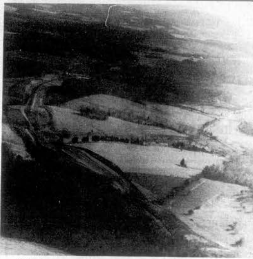
HIGHWAY 72 CONSTRUCTION —This is one of three sections of relocated Highway 72 construction underway in Loudon County. Portions of the highway are being re-located due to the Tellico Lake project and is expected to be complete early next year. This photo was taken near the Harrison family farms in the Southeast section of Loudon County.
