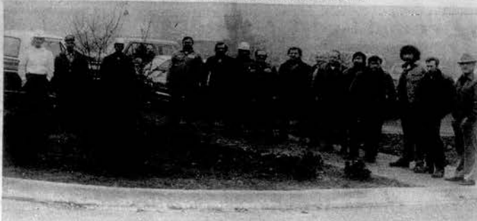
PARKING LOT COMPLETED —A new parking lot for the courthouse, at the site of the old county jail was recently completed. Workmen from the county and city of Loudon
