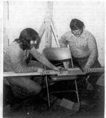
GLENN ROBINSON, INSTRUCTOR for sensory motor activities, and Mike Idorn, vocational occupational instructor, claim credit for many of the recreational props at the center. Besides the chinning frame shown, the two are responsible for the construction of a shuffle board and various games, a balancing beam, tables and bulletin boards used in the center.
