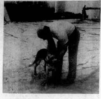
VOCATIONAL SCHOOL Director Coy Gibson greets a dog who has watched every step of construction at the new County Vocational Center. Part of the high-bay area of the school is visible in the background.
