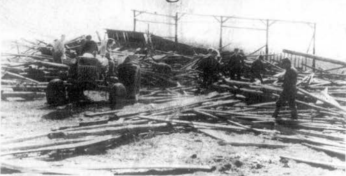
STORM AFTERMATH —A large 90 by 72 barn on the Clarence Bettis farm was completely destroyed in a spring wind and rain storm about 1:40 a.m. Sunday. All but two of the 28 cattle in the barn managed to escape death when the barn collapsed. Debris from the barn was found as much as a half-mile away.
