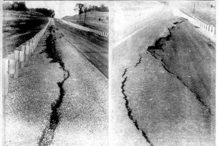
NEW ROAD CRUMBLING —A section of the just completed Sugar Limb Connector is crumbling. Soon after the road was blacktopped around the first week of September a section of the road near the Interstate on a large fill began to crown with the fill crumbling. Rains since have caused major cracks and sags in the road at the fill. A heavy storm last week further weakened the
