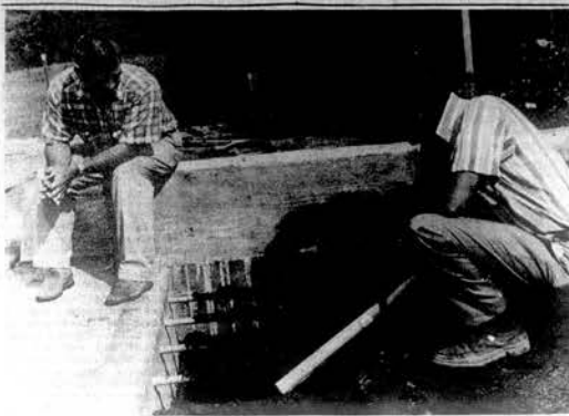
SOIL CONSERVATION SERVICE employees Roy M. Brooks, left, and Fred Carter, right, inspect the manure holding tank after construction was completed recently at Sweetwater Valley Farm.
