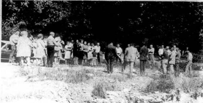
FORK CREEK GROUND BREAKING —Members of Fork Creek Baptist Church are shown at the site of their new church for a ground breaking service Sunday. The new church will be located just off Wade Road. The basement and footings of the church building are visible in the foreground.
