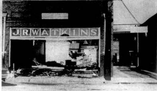
LANDMARK COMING DOWN—For nearly three quarters of a century the Watkins Building on Wharf Street has housed either a grocery-generals store or doctor office. The building was purchased by the Hamilton Bank about six years ago. Recently Dr. J. R. Watkins moved his offices across the street and the bank has started tearing the old building down. The space will be used for a banking remote drive in window and parking lot.
