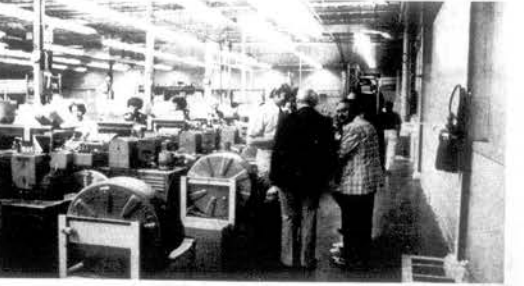
WATCH SHEARING OPERATION—A group of guests touring the Carbide plant stop to watch the shearing operation where casings for "hot dogs" are placed on sticks for shipment to meat packers.
