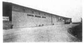
Carter Builders Supply
