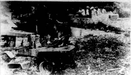
HIGHLAND PARK HOME BURNS —Only a portion of the brick walls and the charred remains of the Bill Issac's family home remained Monday morning when this picture was taken. Friday night a blaze in the basement of the house was extinguished by the Loudon County Rescue Squad. The family was out of town on a Wagon Train ride at the time. About 2:22 a.m. Monday the Squad fire fighters were called back to the house, located at Highland Park. This time the structure was destroyed. The family had been staying in a motel and was not at home. The cause of the fires was not determined. The home and all its contents were a total loss.
