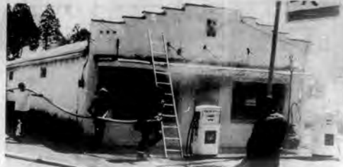
STORE HIT BY FIRE —fire damaged the Hilltop Grocery on Grove Street in Loudon about noon Sunday. Loudon firemen are shown laying hose to battle the fire. The store sustained both fire, smoke and water damage. The building is owned by Carl Gilles. The store is operated by Ronnie Bivens.
