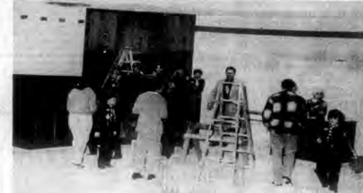
JUSTICE CENTER COURTROOM—Chief Deputy Luke Bright and Civil Defense Director Don Gagley are shown in the courtroom of the new Justice Center with a group of Cub Scouts and their leaders on a tour of the facility Saturday.
