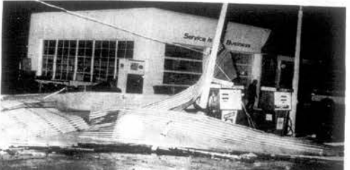
METAL ROOFING CLUTTERED UP MANY BUSINESS AREAS in Lenoir City after the storm. This picture is at the Broadway Shell station.
