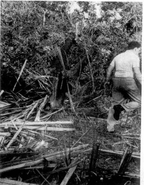
AT BLAST SITE—Two large power poles that once carried two 69,000 kw lines of power to Union Carbide are shown lying in the trees after they were dynamited Wednesday night. The stumps of the two poles and the scattered debris are being inspected by Chief Deputy Lake Bright.
