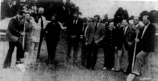
GROUND BREAKING—Mayor Gene Lambert and Health and Education Facilities Board Chairman Ray Birkholz turn the first shovels of dirt at the ground breaking for the 90 bed Care Inn Nursing Home at Loudon last Friday.
