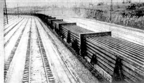
NEARLY 15 MILES of welded, jointless rail moves from Southern's central rail-welding plant at Inman Yard, Atlanta, on a special train developed by the railway's operating department. The six-quarter mile lengths will soon arrive in Loudon County to replace a section of Southern track to provide smoother safer travel in the area.
