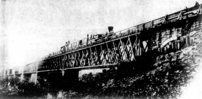
LOUDON RAILROAD BRIDGE (Loudon side) during its rebuilding by Federal troops in 1863. Note the troops in uniform. The bridge had been burned by the Confederates a few months before.
