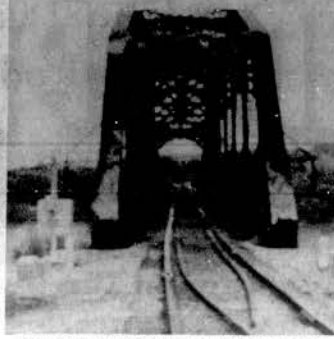
RAILROAD BRIDGE TODAY—The steel structure of the railroad bridge replaced the old wooden structure in 1905 and has not changed in the past 68 years. The rock foundation approaches to the bridge are the same as they were when the bridge was originally built in the mid-1800's.
