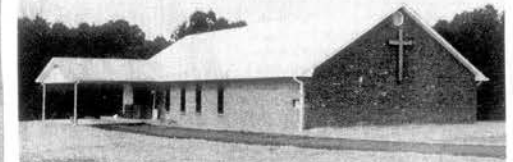
THE BRICK EXTERIOR of the new St. Thomas The Apostle Catholic Church is marked by a simple cross. A covered entrance leads to a paneled narthex which gives pause before entering the sanctuary.
