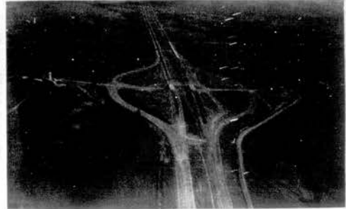
PHILADELPHIA INTERCHANGE —Grading is completed and paving is slated soon at the Philadelphia I-75 interchange shown above. The interchange and section of I-75 is scheduled for completion in May of next year.
