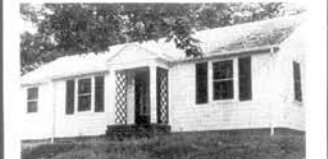
WOULD YOU LIKE to be away from city noise and have enough space for a garden? See this home on River Road in Loudon!!
