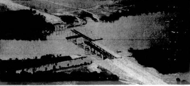
**CLOSING OF THE 1-75 BRIDGE** across the Tennessee River at Loudon is nearing. This aerial photo taken last week shows steel about three-quarters away across the \$7 million bridge. Decking is shown on a portion of the structure.
