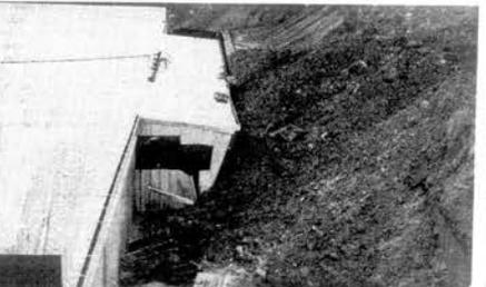
**WALL GIVES WAY**—A retaining wall behind the Cas Walker Store at Lenoir City gave way during heavy rains Friday sending a mud slide into the back of the store, heavily damaging the store and forcing it to close until repairs could be made.
