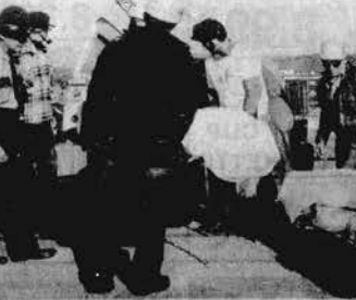
BODIES REMOVED —Workmen on the I-75 bridge construction project at Loudon are shown helping load the bodies of two brothers into a Rescue Squad ambulance shortly after they were killed when a newly poured bridge pier in the river collapsed.
