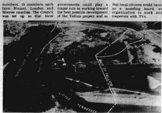
BEFORE... Lines superimposed on this aerial photograph made before construction was started on Tellico Dam, shows the location of the new dam in relation to the existing Ft. Loudon Dam (upper left) and the Tennessee River mainstem. The broken line shows the Z-shaped centerline of Tellico Dam, starting at the south end of Ft. Loudon and running westward (toward the bottom in this photo) across the plain and across Bussell's Island in the Little Tennessee River. The solid white lines show the shoreline of the new reservoir behind Tellico Dam. At upper right is the site of the canal which will link the new CCC reservoir with Ft. Loudon reservoir, diverting the flow of the Little Tennessee River through Ft. Loudon Dam and allowing barge travel on the new lake.
