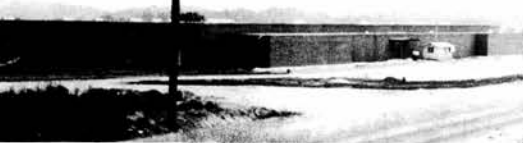
STRIKE DELAYS COMPLETION —Except for work by carpenters and concrete finishers the new Charles H. Bacon Hosiery Company plant in the Loudon Industrial Park is complete. The new 800,000 square foot building will house the finishing and shipping departments of the Loudon mill and will employ some 300 persons when in full operation, hopefully by November 1.
