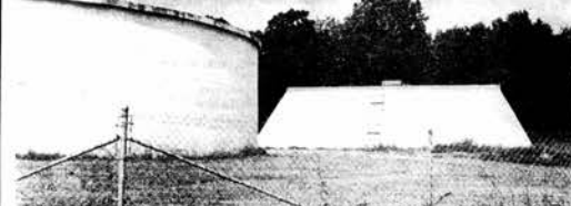
HALF OF WATER STORAGE —These two water storage tanks, 200,000 gallons each on Highland Avenue represent half of the cities reserve water supply. A new 500,000 gallon water tank will be constructed along with a new water treatment plant to give the city 1,300,000 in stored water.
