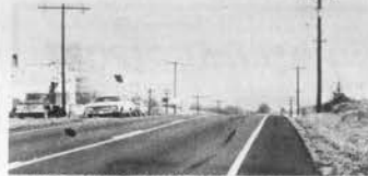
PHILADELPHIA INTERSECTION UNMARKED —Just over this grade on north bound U.S. 11 is an unmarked dangerous intersection leading to Philadelphia. It is the scene of many accidents and some have claimed lives in recent years, but still is not adequately marked.
