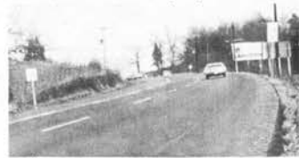
TWO LANES AHEAD —The lone marker at the top of north bound lane on U.S. 11 just out of Loudon on the three lane is not visible to most motorists passing slower traffic going up the hill. Many near crack-ups occur here daily.
