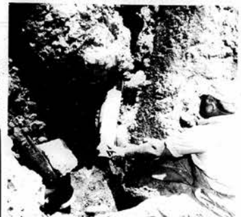
DRAINAGE LINES—Sid McCauley, of the Greenback Community, laying tile for drainage of land on the Mel Hamontree farm. Better use may be made of the land.
