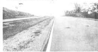
95 AND 11 JUST OVER HILL —Just over this hill on highway 95 is the busy intersection of U.S. 11 (Broadway) at Lenoir City which handles an overload of traffic. Adequate warning signs and signals are absent, thus many accidents at this steep grade intersection.
