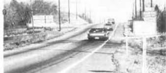
BLIND TO STOPPED CARS —On north bound U.S. 11, two and one half miles from Loudon is the much used intersection with Harrison Road used by many motorists as a route to I-75. Motorists north bound are unaware of cars stopped to turn left across the highway just over the hill. Needs additional marking.
