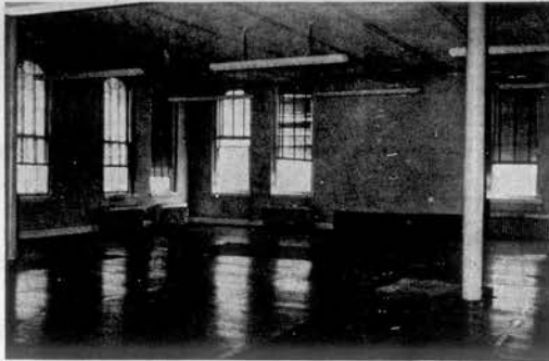
COURTROOM STRIPPED —All the old benches, jury box, and judges bench in the courtroom of the Loudon County Courthouse were stripped out this past weekend to make way for a $55,000 renovation project. The overall size of the courtroom will be reduced as a jury room and judges chamber will also be constructed. The rooms will be air conditioned and have new modern furnishings. Until completed all local court will be held in the General Sessions Courtroom.
