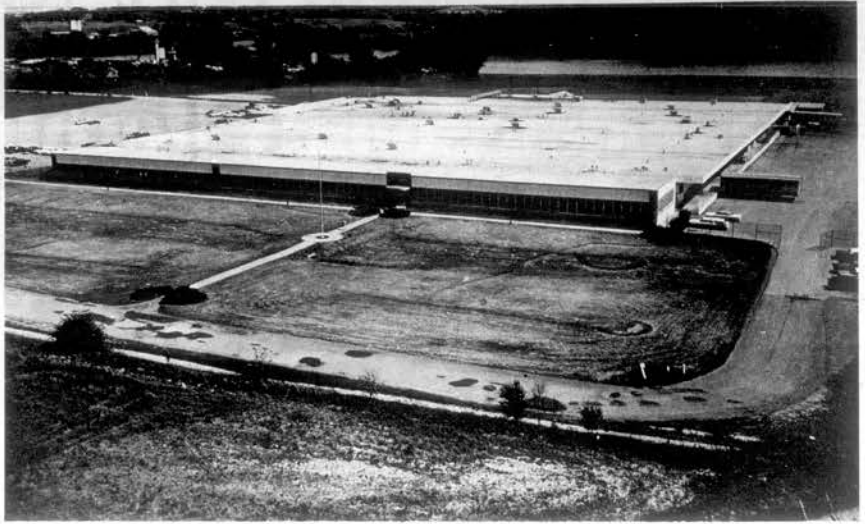
EATON YALE AND TOWNE PLANT IN LENOIR
