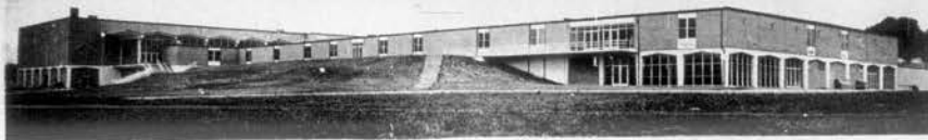
BACK VIEW OF NEW LOUDON HIGH SCHOOL
