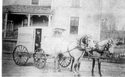
THE DAIRY MILK WAGON of J.W. Bussett about 1909 or 1910 with Charles M. Gassaway as driver. The picture was believed to be taken in front of the John Eldridge home on Kingston Street and Third Avenue. The cows were milked early every morning, the milk prepared and placed on the wagon for deliveries that day.
