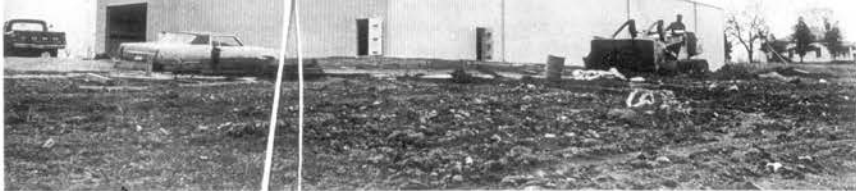
CONSTRUCTION UNDERWAY ON MUNSEY PRODUCTS
