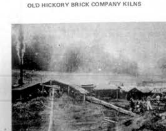
SHOWING THE OPEN AIR dryers in the early days of the Old Hickory Brick Company. About 15 men were employed in the beginning and at its peak employed 40 to 45. Joe Thompson and Jim Dixon are shown with the mule teams for the drag line and clay.
