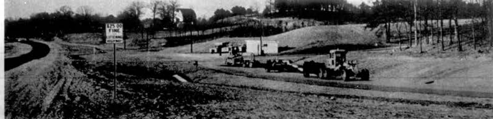
NOT A SMART MOVE—With a warning sign about warning in the foreground the new "temporary" quarters of the state highway department crew in Loudon County decorates the background along the old section of U.S. 11 which was recently replaced when the new overhead bridge was built about a mile East of Loudon.
