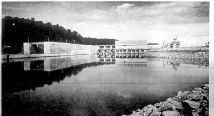
MELTON HILL DAM - TVA's newest dam on Clinch River. The reservoir was impounded in 1963.
