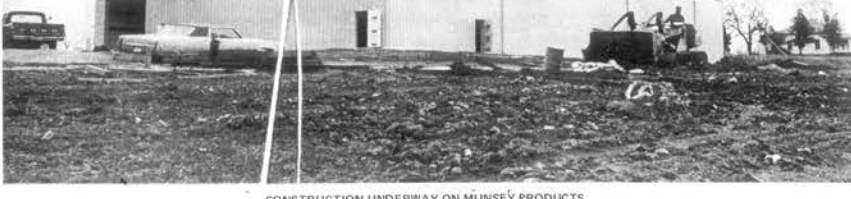
CONSTRUCTION UNDERWAY ON MUNSEY PRODUCTS
