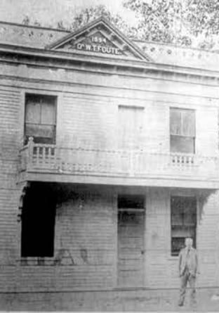
DR. W.T. FOUTE stands in front of the building named after him in Morganton.
