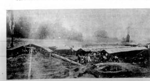
SHOWING THE OPEN air dryers in the early days of the Old Hickory Brick Company. About 15 men were employed in the beginning and at its peak employed 40 to 45. Joe Thompson and Jim Dixon are shown with the mule teams for the drag line and clay.
