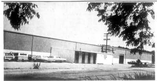
ONE OF NEWEST—Lenoir City's Sheffield Southern Steel Products Co., Inc., located here in 1955. Since then the plant has undergone two expansions to more than double its original size. Starting with 15 workers, the firm now employs about 75.
