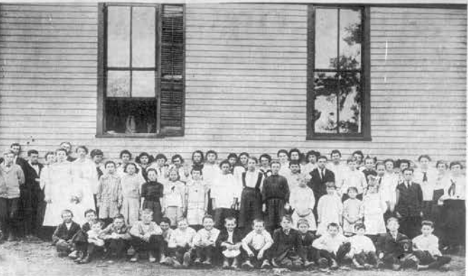
THE OLD BOGART SCHOOL was once a vital part of the educational and community life of the residents of Philadelphia.
